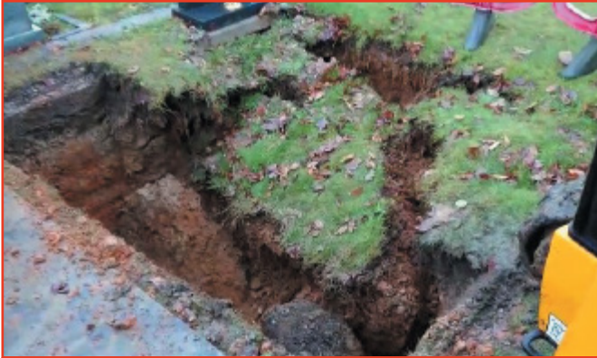
Grave collapse in a UK cemetery
