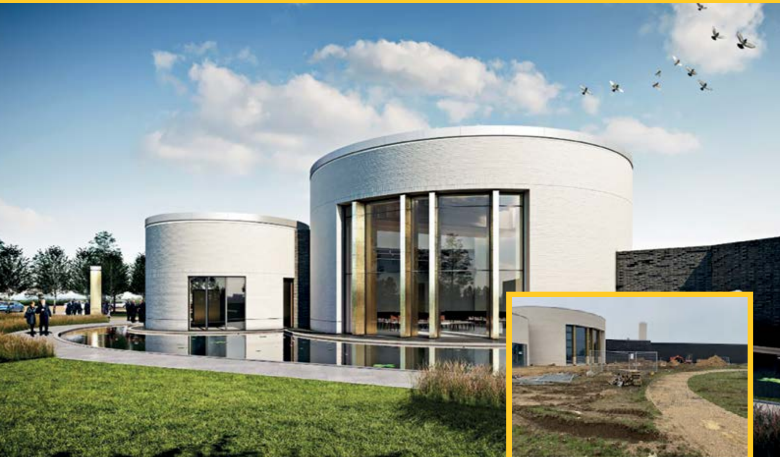
Development in Progress – March 2021
