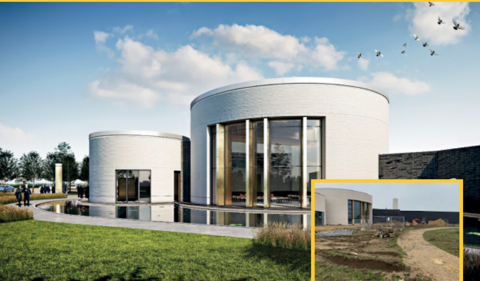
Development in Progress – March 2021
