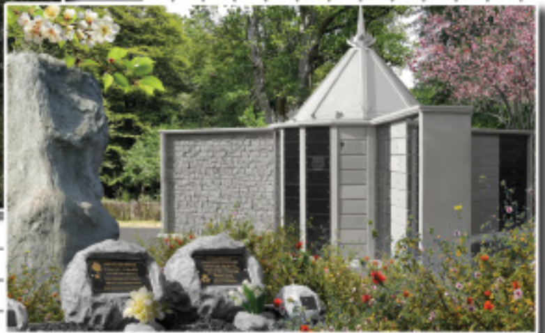
Cremated remains interment provision - installation 2015/19
