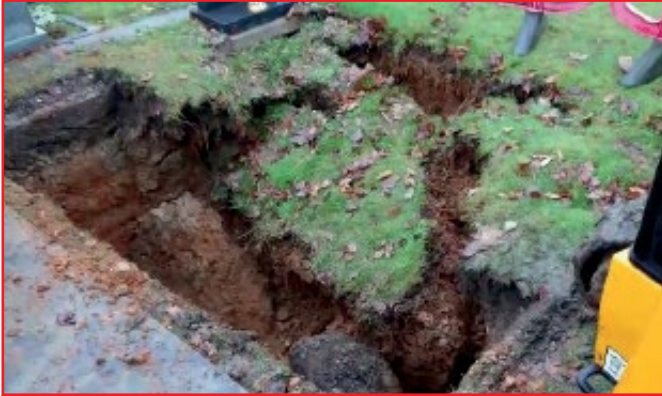
Grave collapse in a UK cemetery
