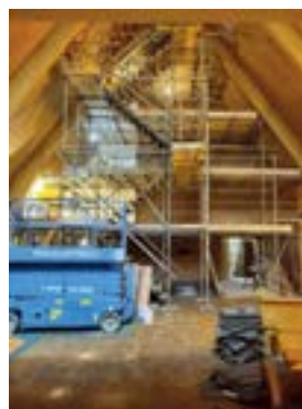
Poole Ceremony Hall – removal of Skylights
