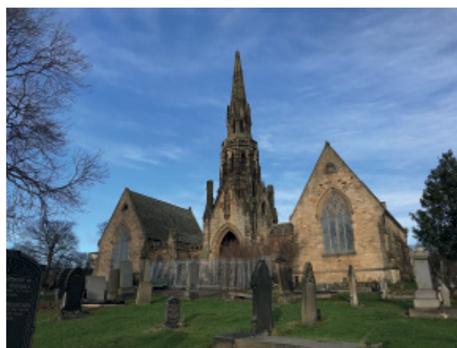
The redundant chapels in St John's Elswick Cemetery (1856) in Newcastle urgently need restoration.
