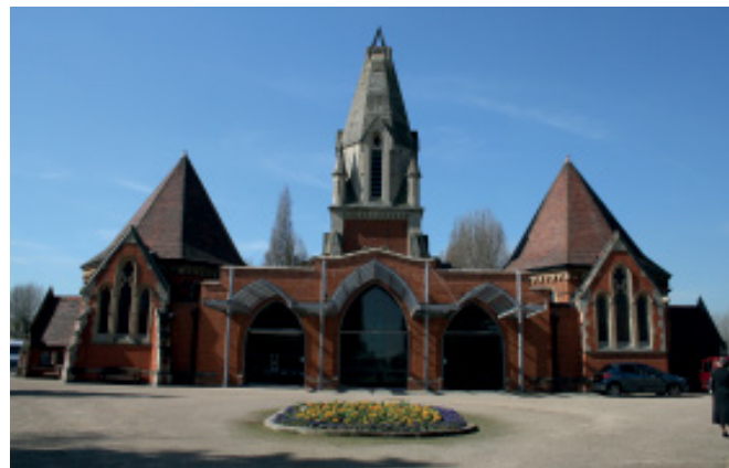
The chapels in Battersea New Cemetery in Morden, Surrey, were converted into North East Surrey Crematorium in 1958.
