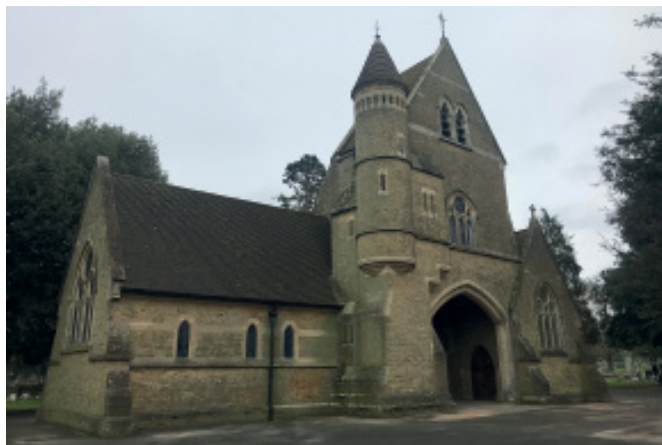
The substantial chapels in Chatham Cemetery (1869).
